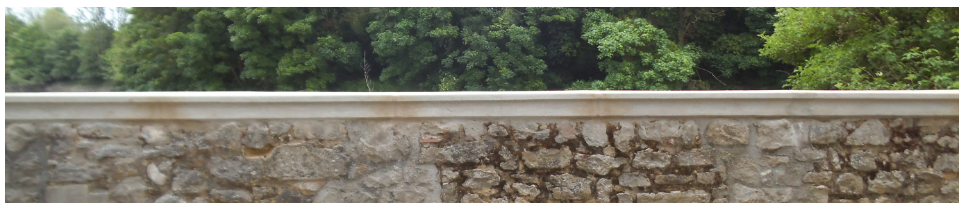
The restored riverside wall, Aylesford
