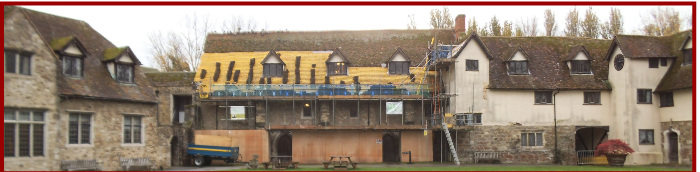
Thirteenth Century Pilgrims' Hall roof undergoing repairs
