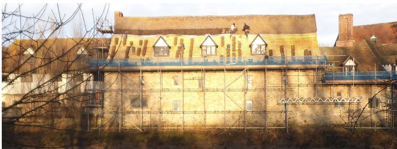
Re-roofing the thirteenth century Pilgrims' Hall (riverside view)
